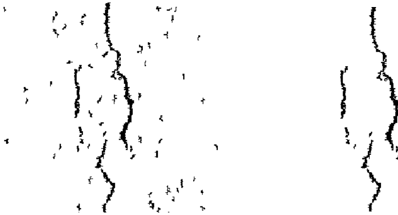
(a) Before Elimination of Tiny Cracks (b) After Elimination of Tiny Cracks
