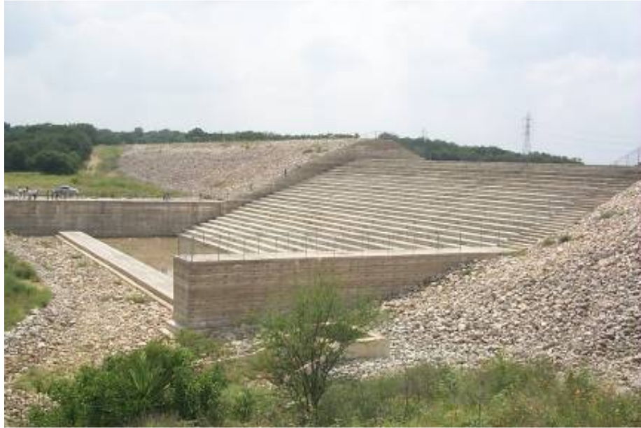
Figure 1.1. RCC stepped spillway on an embankment dam.
