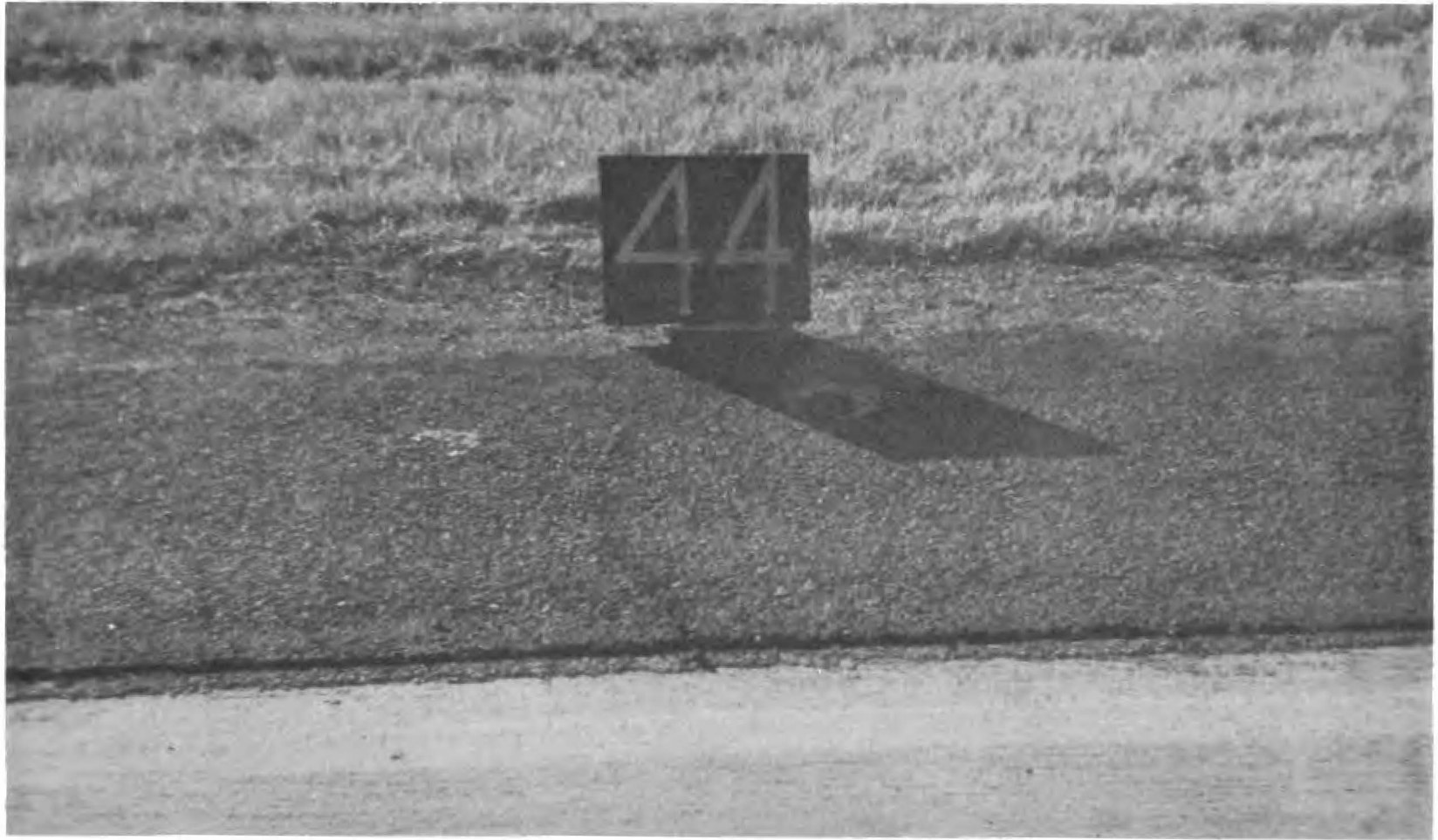
Figure 3.2. Differential Movement of Shoulder at Site No. 44
