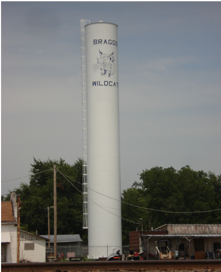
Figure 1.2: Central water tower at Braggs, Oklahoma
