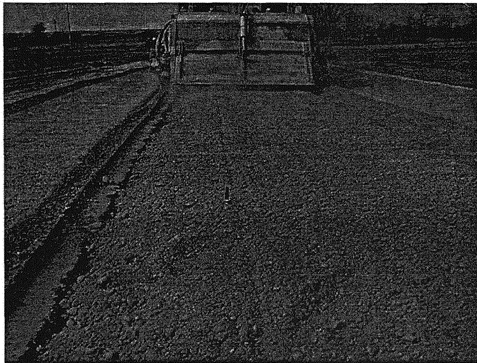
FIG. B-4 Mixing with Bomag Recycler: A) Lime and B) CKD
