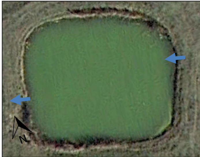
Figure 2-7 Aerial photograph of the VFBR at the Hartshorne PTS. The blue arrows indicate where the water enters and leaves the cell. (Google Earth 2012)
