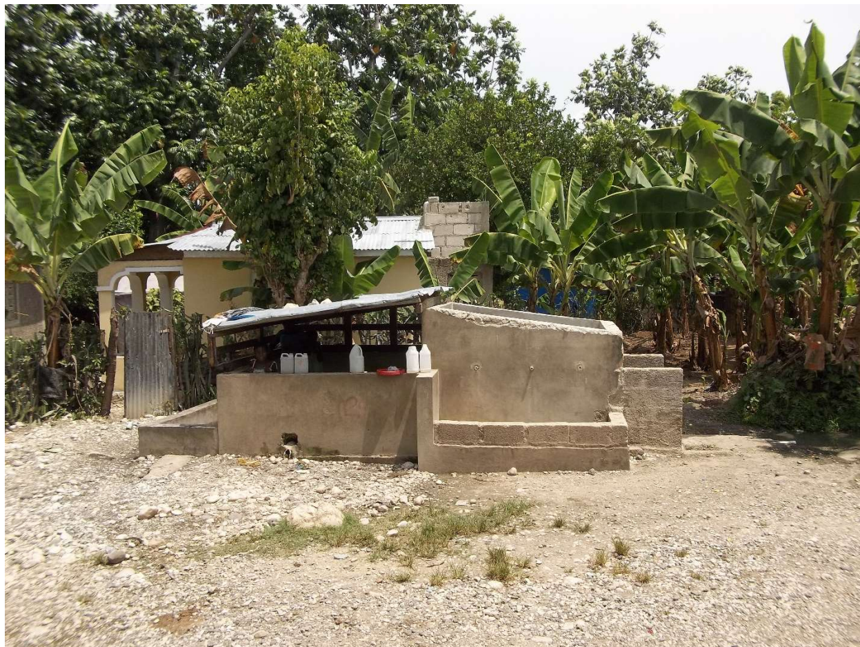
Figure 13: Building constructed around pump
