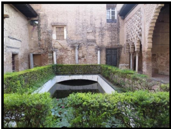
Figure 11: Pool of the Patio del Yeso
