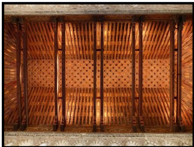
Figure 57: Ceiling detail, Sinagoga del Tránsito
