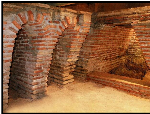
Figure 45: Brick work detail, Santa Clara de Tordesillas
