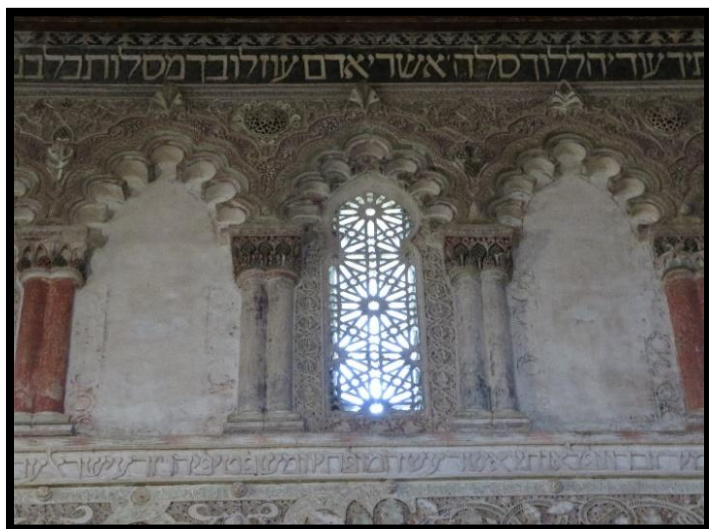
Figure 50: Poly-lobed fenestration detail, Sinagoga del Tránsito
