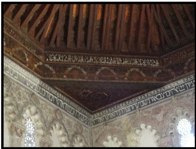
Figure 59: Ceiling detail, Sinagoga del Tránsito
