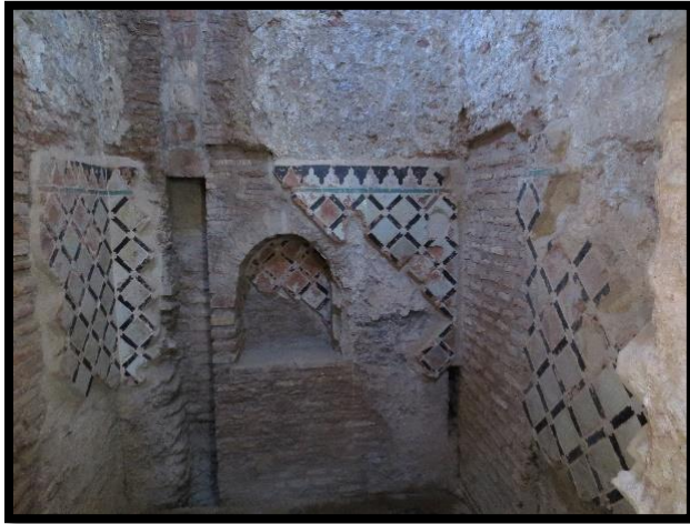
Figure 46: Tile detail, Hammam, Alhambra
