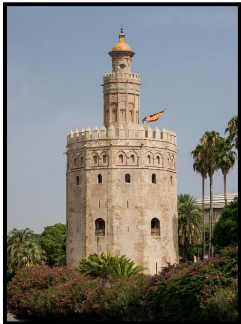
Figure 83: Torre de Oro, Seville
