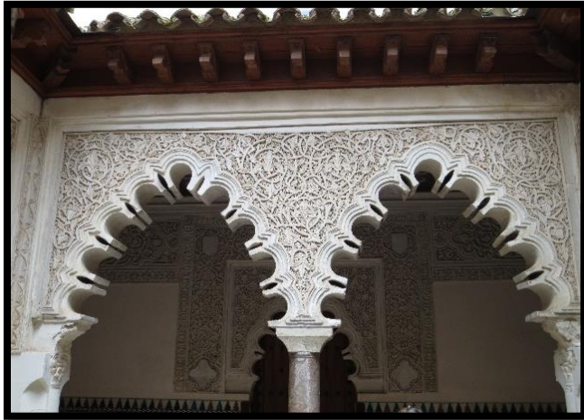
Figure 41: Poly-lobed arch detail, Patio Árabes
