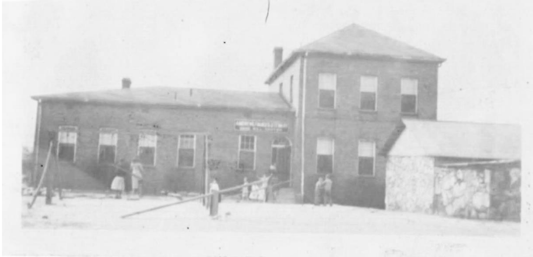
Figure 17 Side view of the Pelham Street location. This building was much larger than the Bellwood Avenue house, and designed specifically with the programs of the Stewart Center in mind. Courtesy of the Andrew P. Stewart Center.
