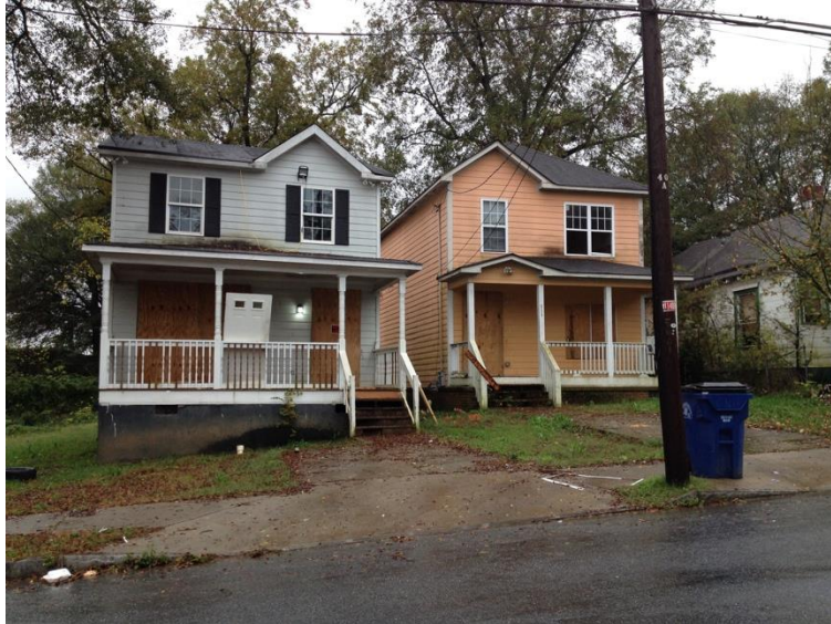
Figure 48 Two houses purchased by the Stewart Center's Pittsburgh Community Housing Program, prior to rehabilitation. 552 and 554 Rockwell Street.
