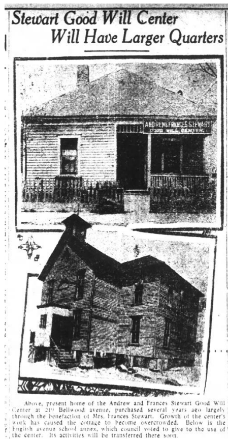
Figure 15 Newspaper article showing original Stewart Center and English Avenue School Annex. Atlanta Constitution, April 26, 1923, page 6.
