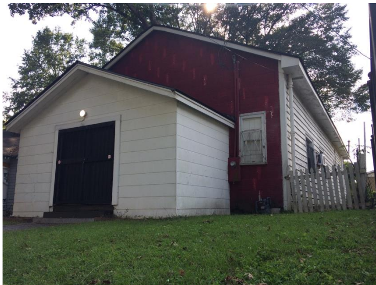
Figure 21 St. James Baptist Church, English Avenue. Originally built as the Chapel-Recreation building for the Stewart Center, the building is still owned by the African American church that purchased it in 1949. Photo by author.
