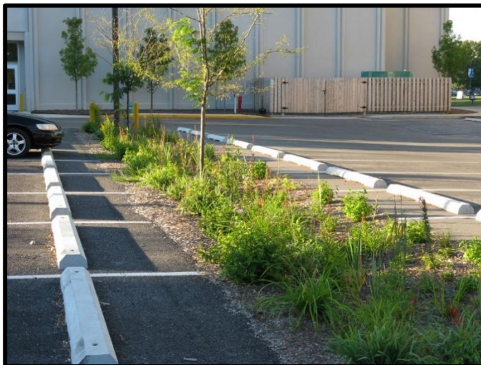
Figure 8. Typical Rain Garden. Source: Butler University
