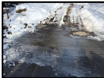
Figure 3: Existing Low-Water Crossing Looking East
