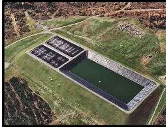
Figure 11: Typical Wastewater Lagoon.
