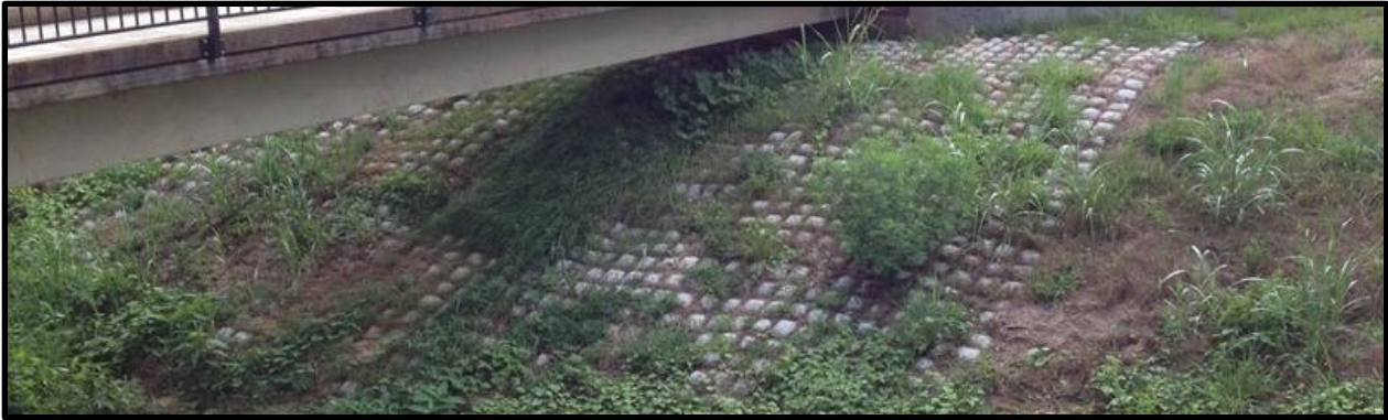
Figure 17: Tied Concrete Block Mat. Source: Brock White Manufacturing
