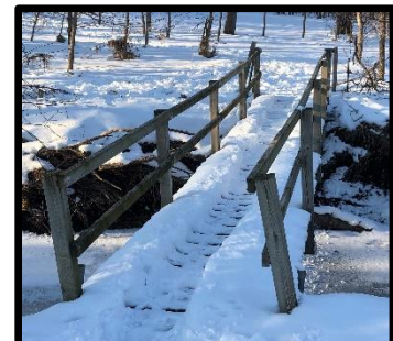
Figure 2: Existing North Scout Creek Pedestrian Bridge Looking Northeast
