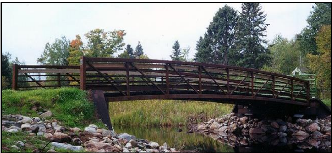
Figure 18: Riprap around Bridge Abutments. Source: Wheeler-Con
