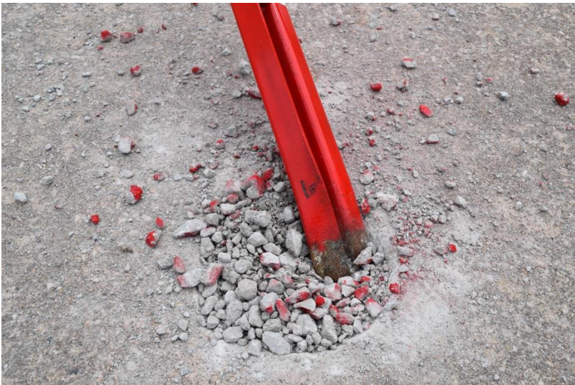
Figure 92. Time-Sequential and Post-Impact Photographs, Test No. MWFPF-19
