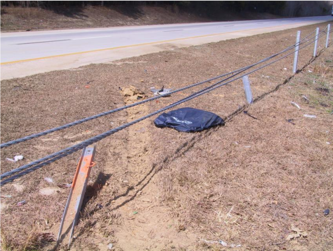
Figure 99. Diving Underride Penetration Crash in North Carolina
