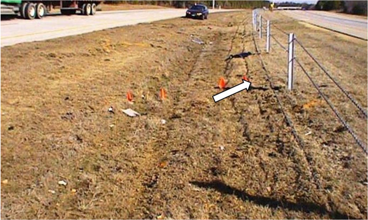
Figure 104. Back Side (Middle) Cable Release from 11 Downstream Posts Resulting in Penetration
