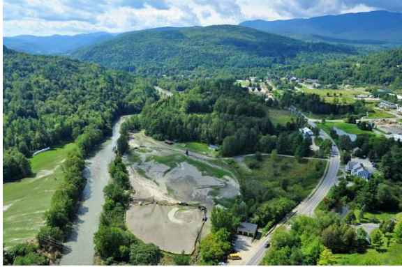
Figure 3. 19. Sediment deposits from flooding.
