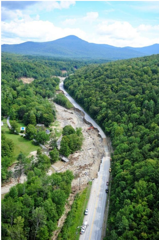
Figure 5.13. Route 4 washout along Mendon Brook, Mendon, Vermont.
