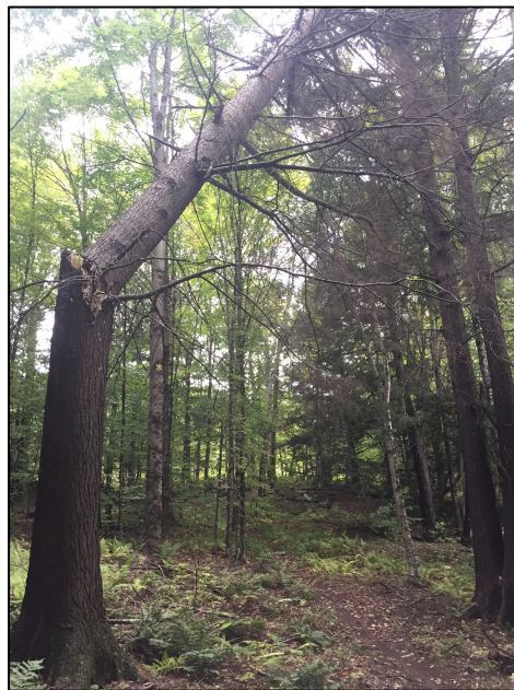
Figure 22: A snapped tree or “widow-maker” hangs over a multi-use trail in Morrisville, VT. Photo credit: Taylor Luneau
