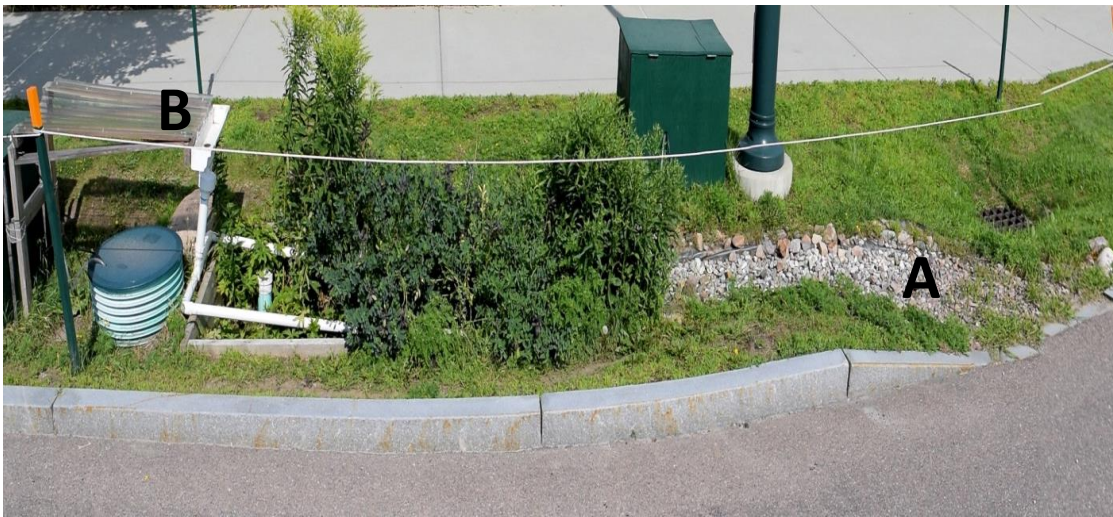
Fig. 1. Bioretention cell at the University of Vermont, Burlington, USA. The cell receives road runoff via curb cuts along the road. (A) Shallow rock-line inflow swale, underlain by high-density polyethylene (HPDE) plastic, conveys runoff into the cell's weir. (B) Rainpan and attached PVC precipitation-distribution pipes. The rainpan is installed outside of the cell. Rainwater from the corrugated pan drains into gutters, vertical downspouts, and to pipes that run horizontally along the length of the cell and contains perforations at the bottom to deliver water evenly across the cell. Photo credit: Lindsay Cotnoir.
