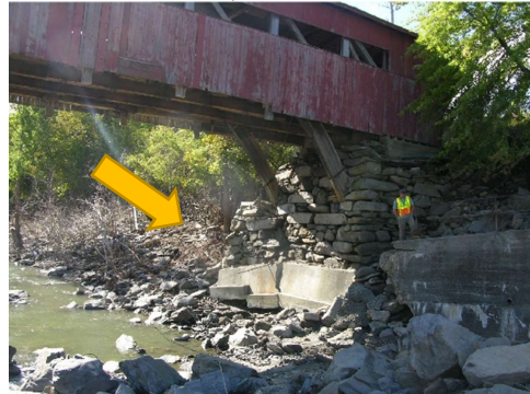
(c) Example of extensive scour damage – before and after, Woodstock C2002 B45
