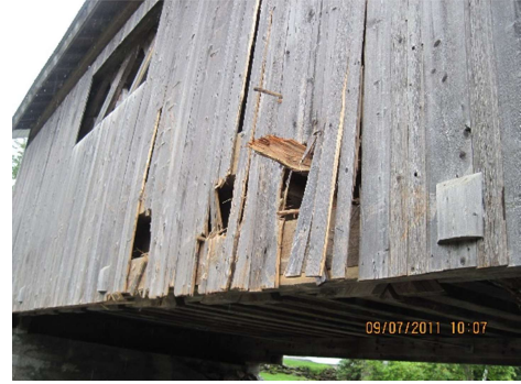
(a) Example of slight debris damage – before and after, Montgomery C2001 B5
