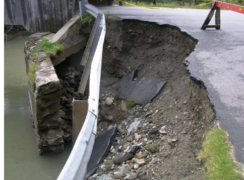
(b) Example of moderate flanking damage – before and after, Warren FAS188 B6
