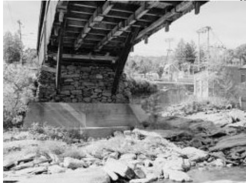
(c) Example of extensive scour damage – before and after, Woodstock C2002 B45
