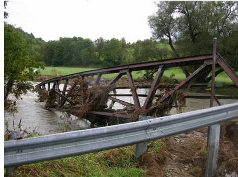
(d) Example of complete damage – before and after, Moretown C3024 B41
