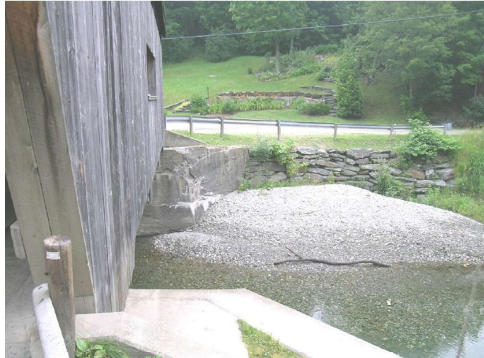
(b) Example of moderate flanking damage – before and after, Warren FAS188 B6
