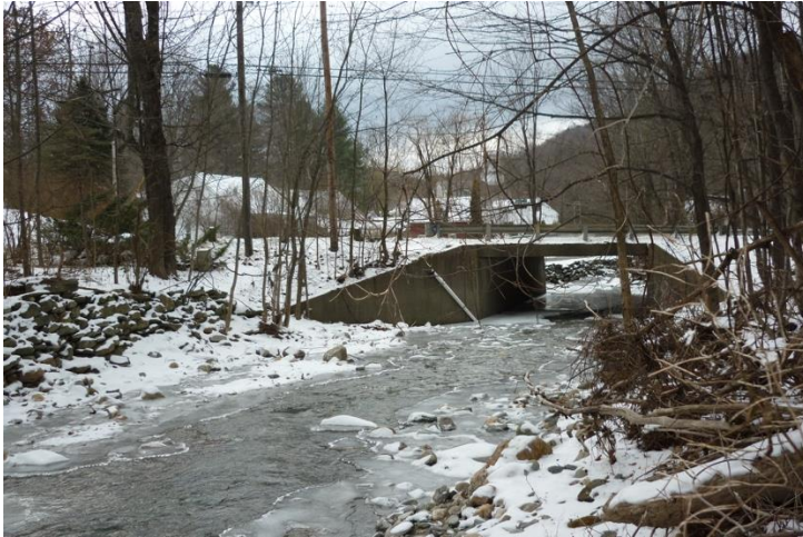
Freeman Brook turbidity sensor and stage sensor installation looking downstream
