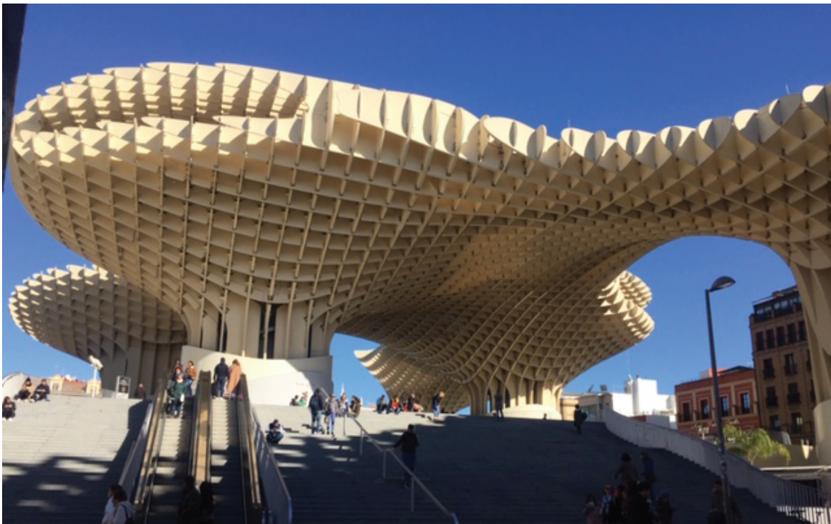
Las Setas, the largest wooden structure in the world.
