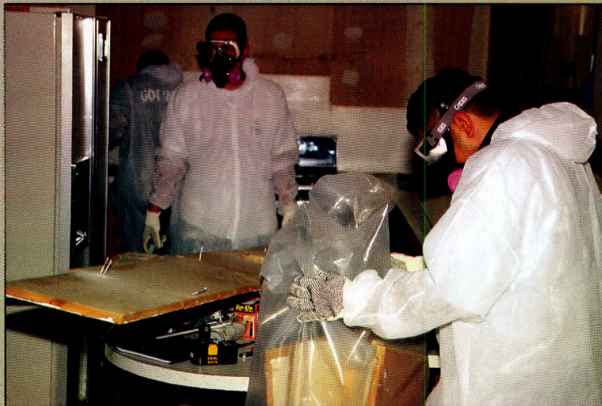
COMMERCIAL REMEDIATION teams follow protocols to remove extensive mold infestations. Most outbreaks can be cleaned using bleach and water.
