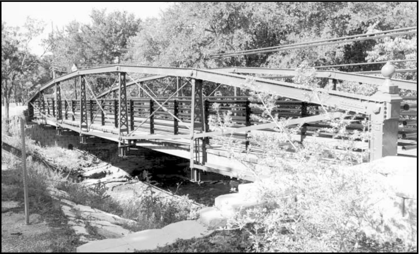
The rare lenticular pony truss bridge relocated from Dodd's Creek and renovated as a pedestrian walkway in Salado.
