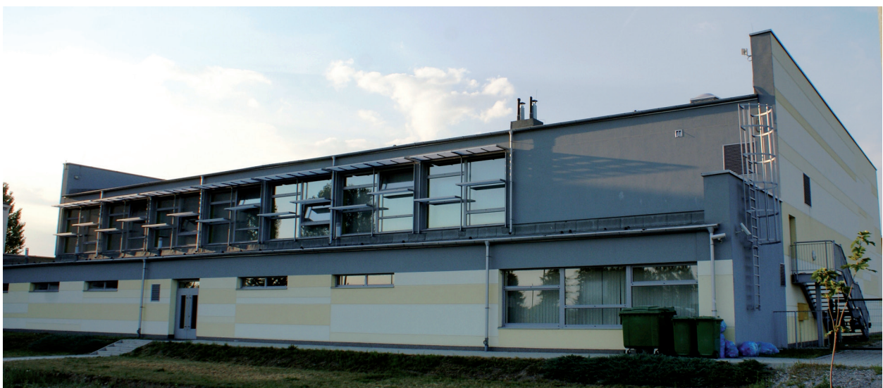
Photo 2. South view of the sports hall at Słomniki (Małopolska), the first passive public building in Poland with a quality certificate awarded by the Passive House Institute.
