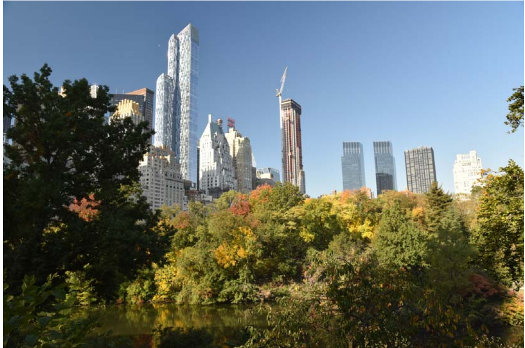
Fig. 7. Southern frontage of the building development along Central Park. In the foreground: One57 (Christian de Portzamparc, 2014). In the background: the construction of 220 Central Park South (Robert A.M. Stern); author's photograph
