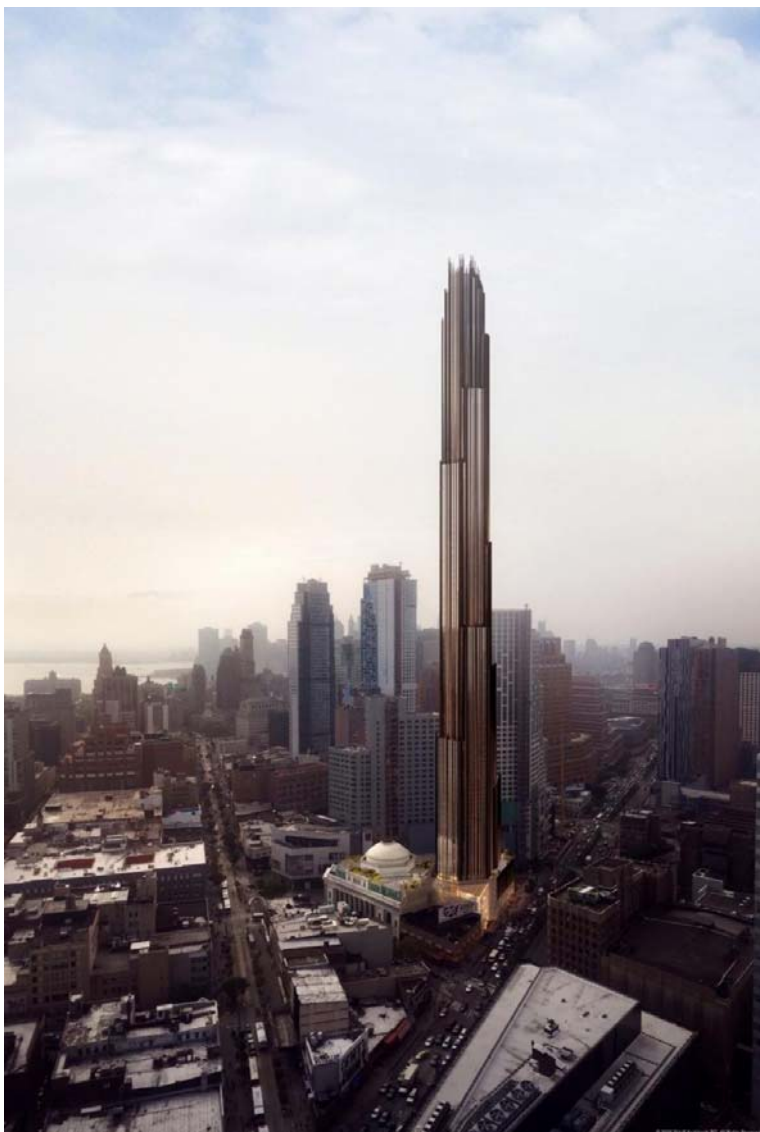
Fig. 12. 9DeKalb building at 325 meters tall, being designed in Brooklyn. Source: [11]
