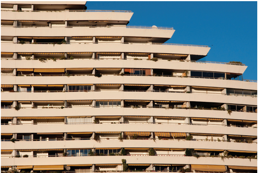
Photo 8. Partial view of a building in Marine des Anges (Villeneuve-Loubet)
