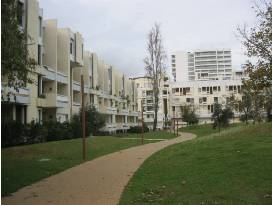
Photo 1. Partial view of the buildings in “Tróia’s Garden City”
