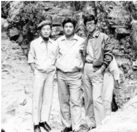
Figure 23 Ch'unch'on Soyang Dam Excavation 1971. Chi Kon-gil, Ku Ch'ol-hui, Ch'oe Mong-nyong. Chi Kǒn-gil, Kogohak Kwa Pangmulgwan Kŭrigo Na: Chi Kǒn-Gil Chǒn Kungnip Chungang Pangmulgwanjang Ŭi Pangmulgwan Hoegorok , 25
