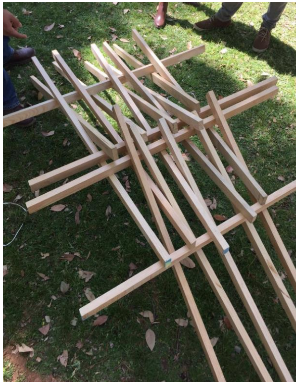
Figure 4 Bridge frame reciprocal structure. Source: Own
