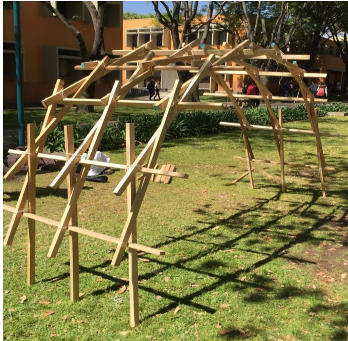
Figure 5 Portal structure of reciprocal frames. Source: Own
