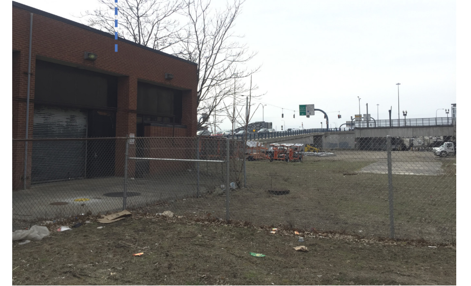
high pressure water pump station
