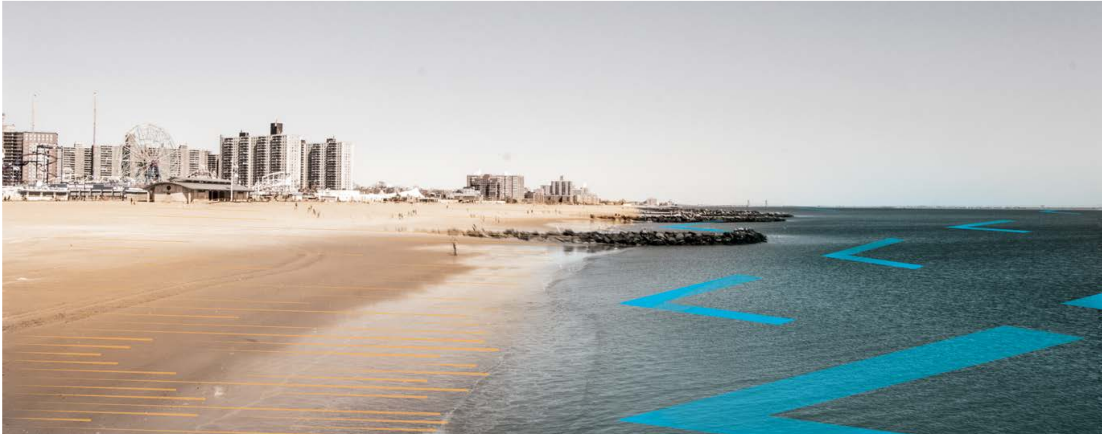
Along the shore, groins have been constructed to slow steady drift of sand down the coast.
