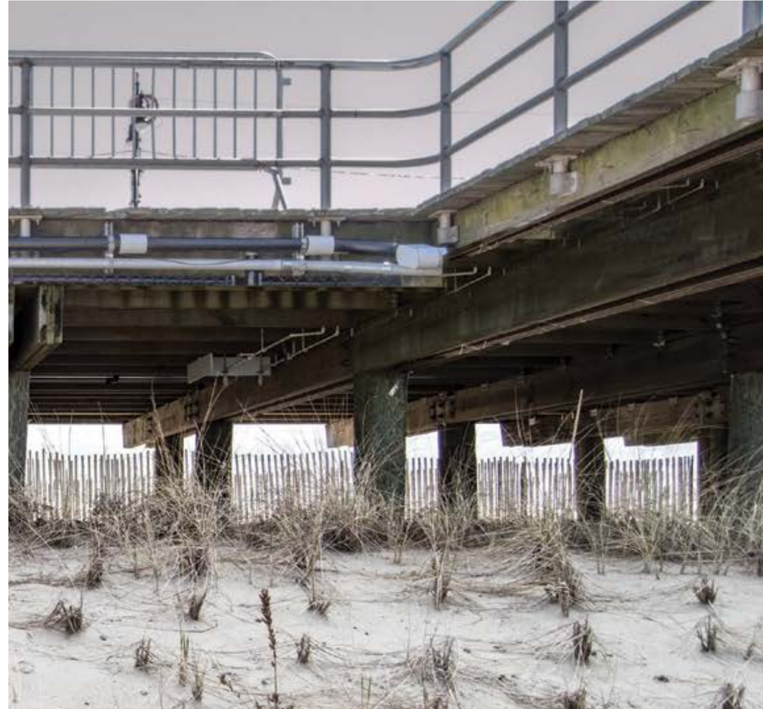
An initial testable solution that emerged was to hybridize the boardwalk with existing dune restorative strategies.
