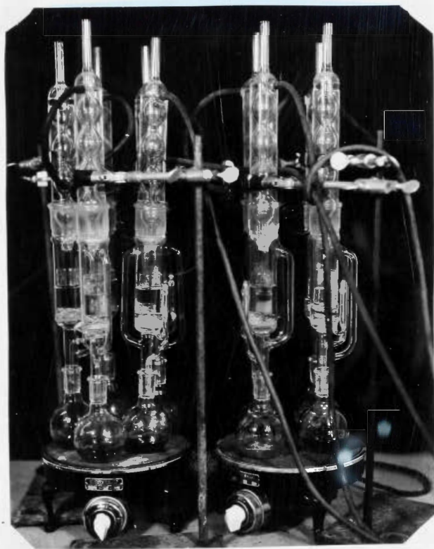
Figure 1. Soxhlet extractor installation used for extracting reducing sugars and sucrose.
