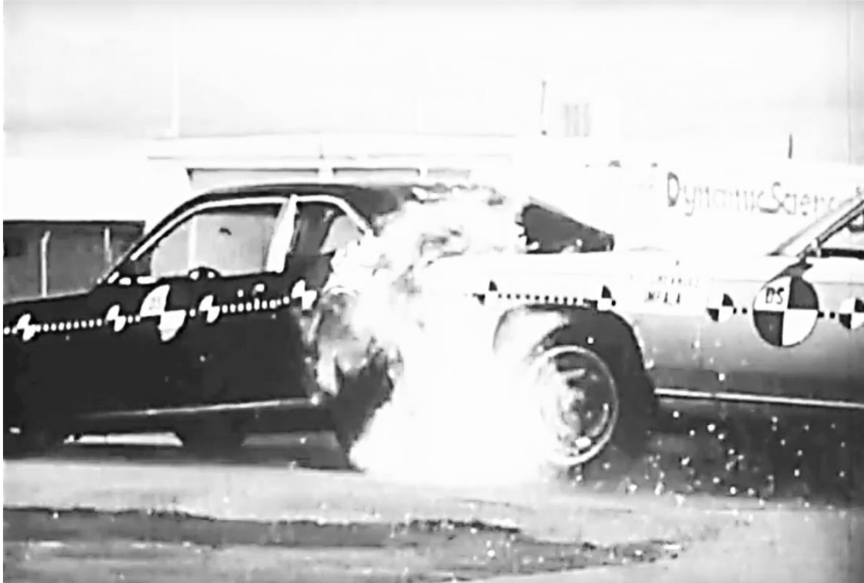
Figure 1. Ford Pinto Fiery Test Crash
