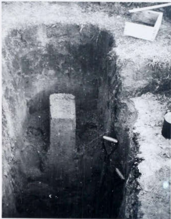
Figure 4. Removal of 8 by 8 inch columns. The first two feet have been removed from the column of soil.
