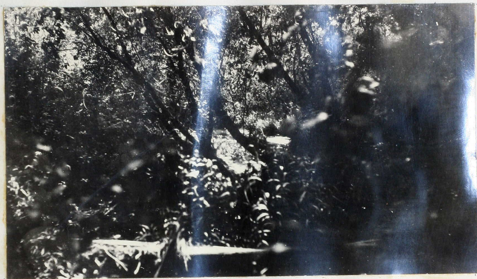
Fig. 6. A small portion of the vegetation covering the lower side of the dam.
