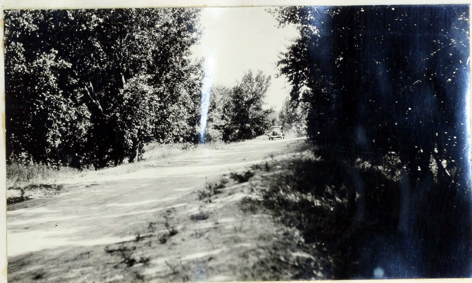
Fig. 4. A view of the dam showing the road formed.
