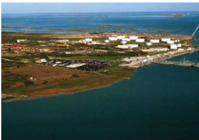
A VIEW FROM ABOVE The base for Naval Station Ingleside, scheduled to close in September 2010, will be redeveloped for renewable energy research by the A&M System under an agreement with the Port of Corpus Christi Authority.
