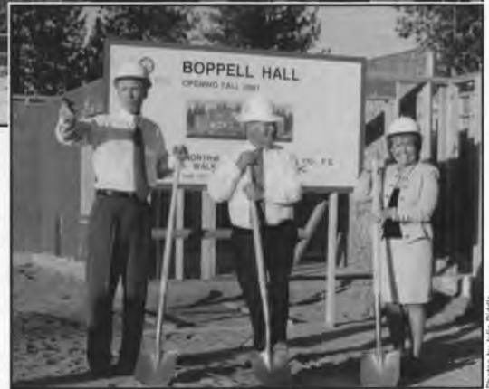
Bill Robinson and Chuck and Karlyn Boppell break ground in April for the building bearing the Boppells' name. At top, Boppell Hall in mid-construction.
