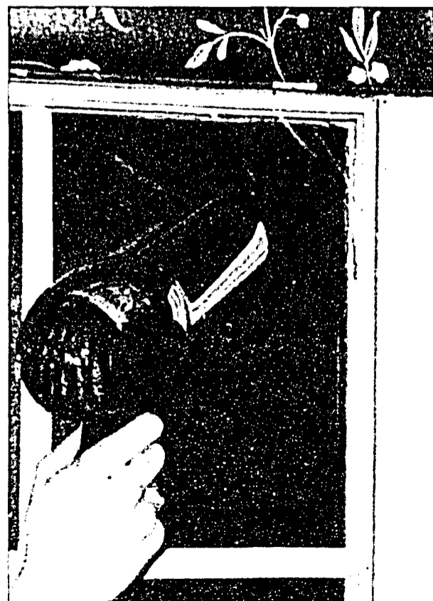
LEFT: Applying insulating shrink wrap to windows cuts down on heating costs.
