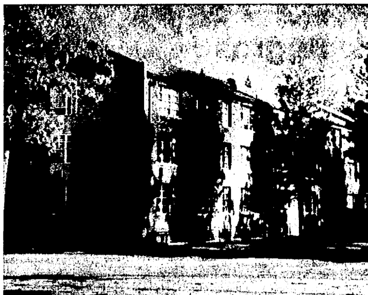
THREE FLOORS OF SPACIOUS BEAUTY. A year of hard labor and cramped quarters will officially be at an end when Whitworth dedicates her new women's dorm, South Warren, Sunday, February 24. The addition is presently being occupied and is connected to the south end of the present Warren hall.
