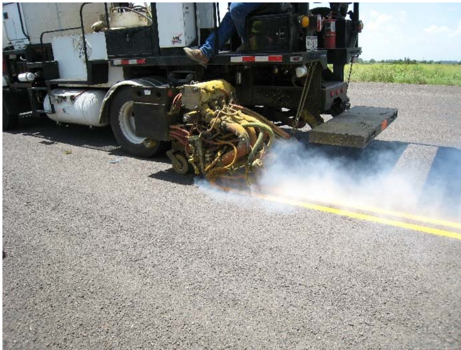
Figure 24. SH 21 Lead-Free Thermoplastic Installation.
