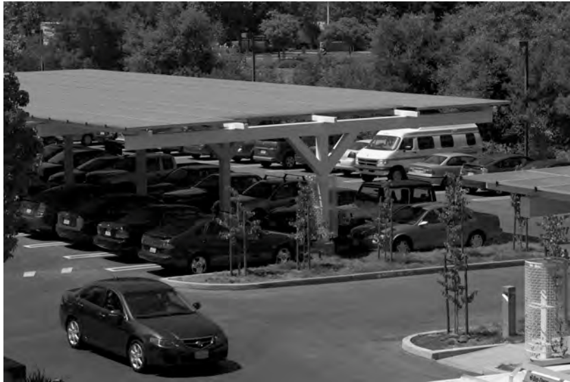
Figure 11.2: © Google, Carport Solar Panels
