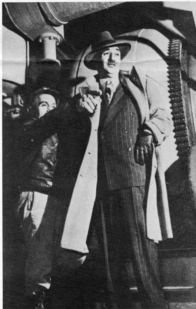
Foreman points out site for new building to Nathan Manilow, Chicago builder, who gambled $1,000,000 bank-rolling the project originally
