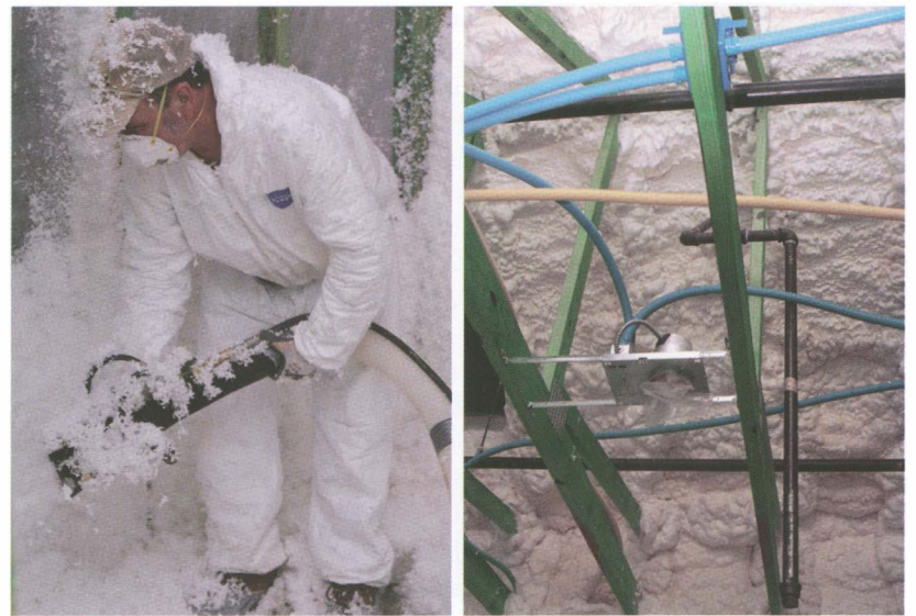
The great room features the work of local artists. The mantle, crafted by John Wicks '09, came from a piece of reclaimed wood. This page, clockwise from upper left: A pre-cast foundation produces less waste and fewer toxins; the specially treated structural framing provides exceptional protection and durability; extensive insulation blown into the walls and ceilings makes for a quieter home, improves air quality and protects against air leakage, moisture and airborne allergens. All photos by Jeremy Fleming except where noted.
