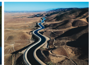
Irrigation canal in the desert
