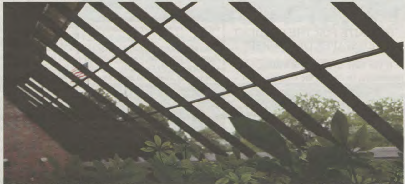
D-Wing foyer inside the main entrance of GSU.
