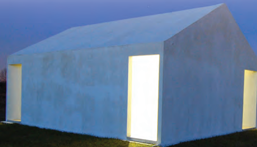
House Divided 1983 Bruce Nauman cast concrete Commissioned by the GSU Foundation, Nathan Manilow Sculpture Park 1983.02
