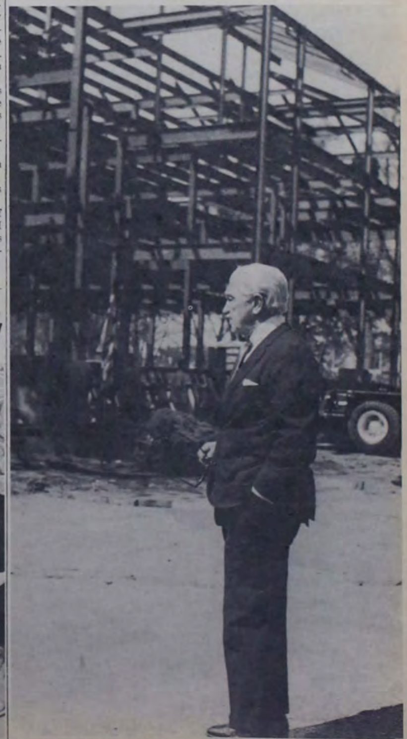
Former President Helfferich surveys the progress of the construction of the new Myrin Library during the final days of his administration.
