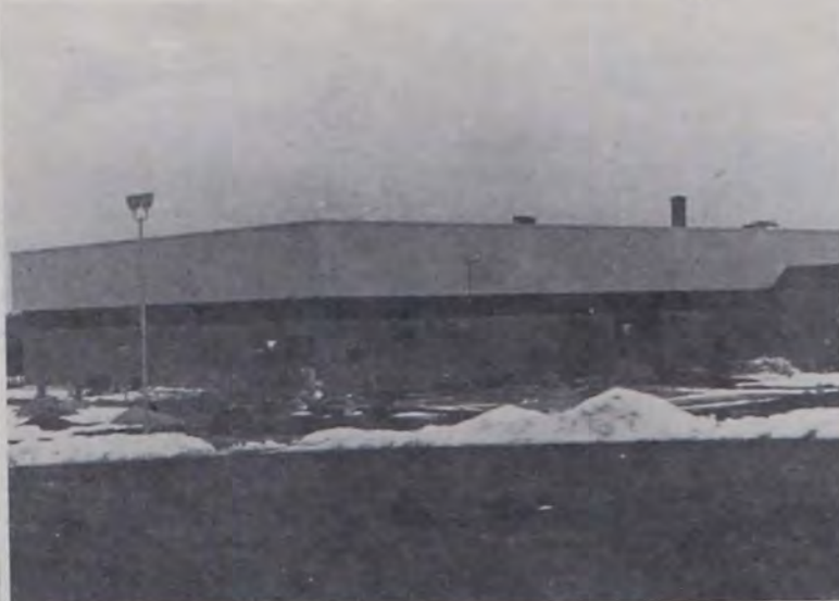
New Gymnasium facilities almost complete.
