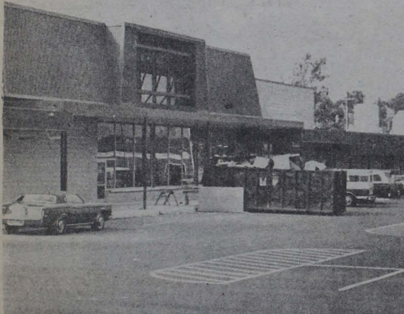
Work continues on main building.
