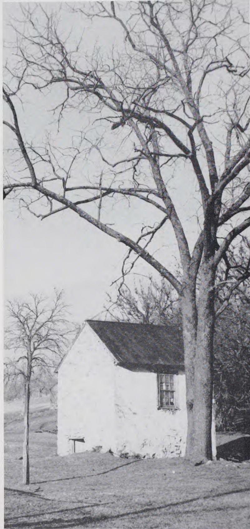
Many spring-houses had two levels for refrigerating different foods. The first floor of this one was entirely below the ground level and was doubtless used for cooling dairy products such as butter and cheese. The second floor was available for storing vegetables or other foods which needed less refrigeration.
