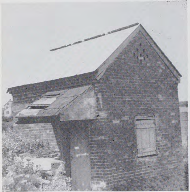
This mid-nineteenth century spring-house is located in southern Lancaster County. Its architectural features are similar to the farm house which stands nearby. The serrated brick cornice is typical of the time and area. There is little provision for light in any of these spring-houses.
