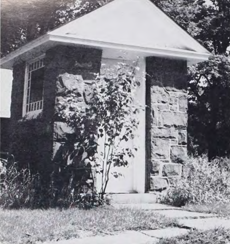
BROWN SANDSTONE PRIVY WITH STAINED GLASS WINDOW. This well-built structure is located on the property of Erma J. Walton, Route 3, Hummelstown. Dimensions: 7 ft. square, 7 ft. high. Photographed 1962.
