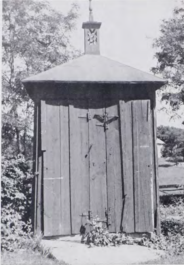
DOUBLE PRIVY. Notice construction of hardwood boards with battens, double doors and ventilating lower. Located on Paul H. Martin Farm, Route 5, Lebanon. Dimensions: 6 ft. square, 8 ft. high, to lower. Photographed 1962.
