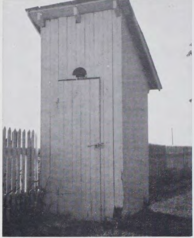
MENNONITE MEETINGHOUSE PRIVY. Located on Mennonite meetinghouse property in South Lebanon Township on road leading from Cornwall to Schaeffers-town. Dimensions: 4 ft. square, front 10 ft., rear 7 ft. Note vent above door. Photographed 1962.
