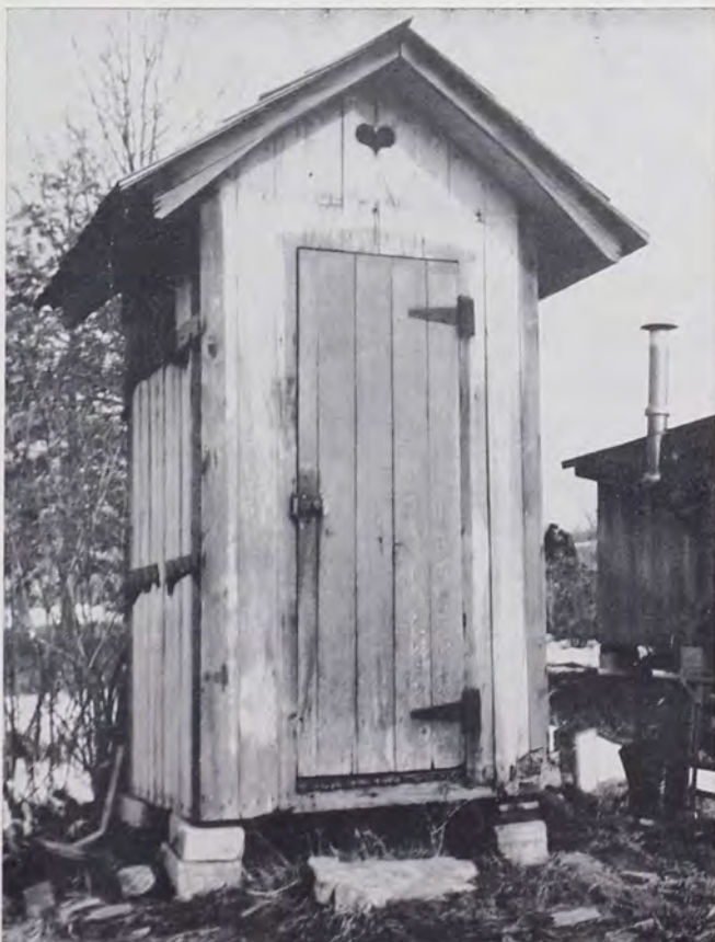
PORTABLE PRIVY WITH PENNSYLVANIA DUTCH HEART MOTIF. Located on property of Ivan Fasnacht on Route 897 between Schaefferstown and Kleinfeltersville. Now used for gas and oil storage. Dimensions: approximately 4 ft. square, 8 ft. high. Photographed 1962.
