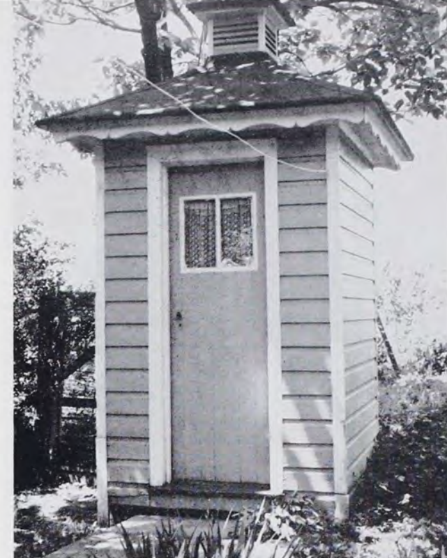
WELL-KEPT CONTEMPORARY LEBANON COUNTY PRIVY. Note curtains on window, lowered ventilator-turret, scalloped roof edges. Located on property of Mrs. Eva Wolfe, Route 1, Lebanon. Outside dimensions: 4'8" square, 7 feet to roof, 10 feet to turret. Double wall construction. Color: bright lemon yellow. Photographed 1962 by Amos Long, Jr.
