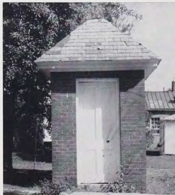
BRICK PRIVY WITH SLATE ROOF. This well-constructed privy, located in Cleona on the northeast corner property, Lincoln and Maple Streets, is now used primarily for storage. Dimensions: 6 ft. square, 10 ft. high. Photographed 1962.
