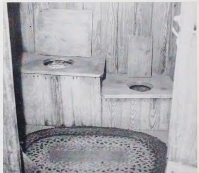
ALL THE COMFORTS OF HOME. Interior of Lebanon County privy shows two levels of seats, one at 18 inches for adult, the other at 12 inches for small child. Note oval or egg-shaped holes and lids, hand-braided rug on floor, broom in corner. Interior dimensions: 4 ft. square. Located in rear of 417 E. Main St., Annville, Pennsylvania. Photographed 1963.
