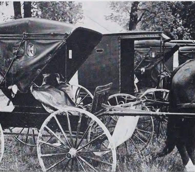
"PLAIN" CARRIAGES AT LANCASTER COUNTY MEETINGHOUSE. These plain carriages are locally manufactured, but follow the traditional lines of the rural American buggies and spring wagons of the pre-world War I era. They are well built, and must be uniform in style. The electric light, powered by batteries, is a state requirement. So hazardous is carriage travel on today's highways that certain counties in Ohio where there are large settle-
