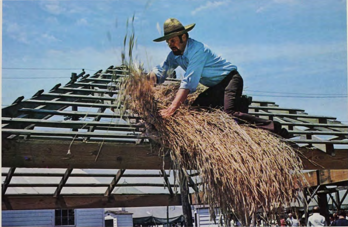
Thatching the hay barrack
