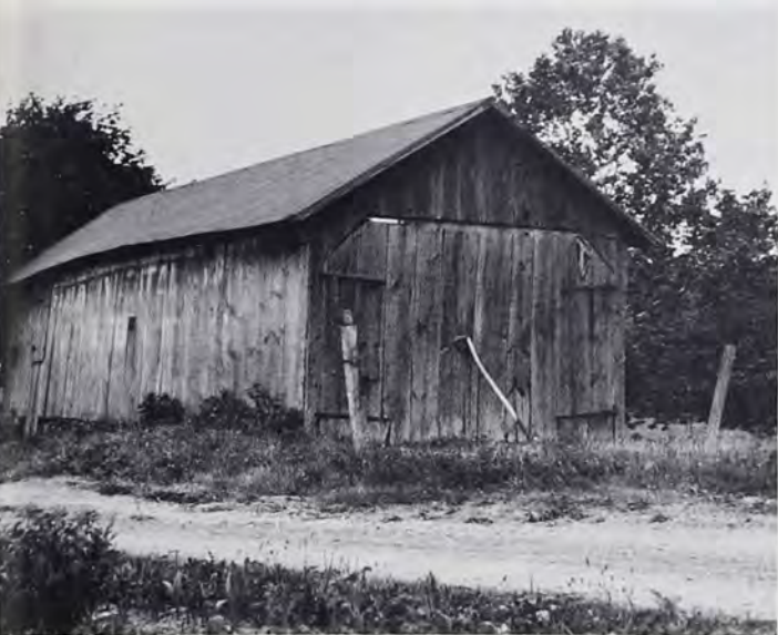
Frame structure near Bernville, Berks County, the left end of which was once used for ice storage.
