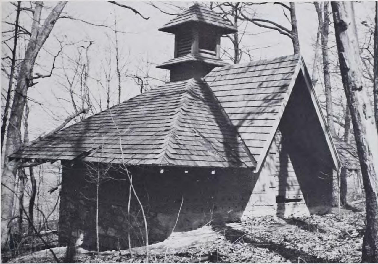
Victorian Ice-House on former Coleman-Altman Estate in Lebanon County. Note ventilating louver, similar to those on fancy Victorian barns.
