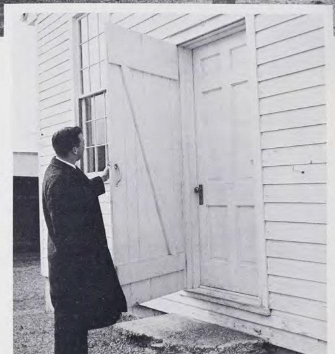
Author examines double door at meetinghouse. The community does its own carpentry work.
