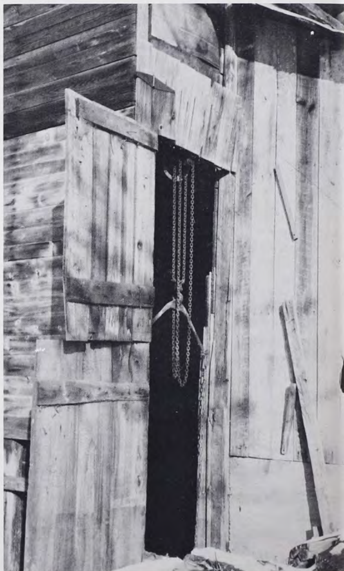
Ice-House Doors and Chain Hoist used to lift ice into building.
