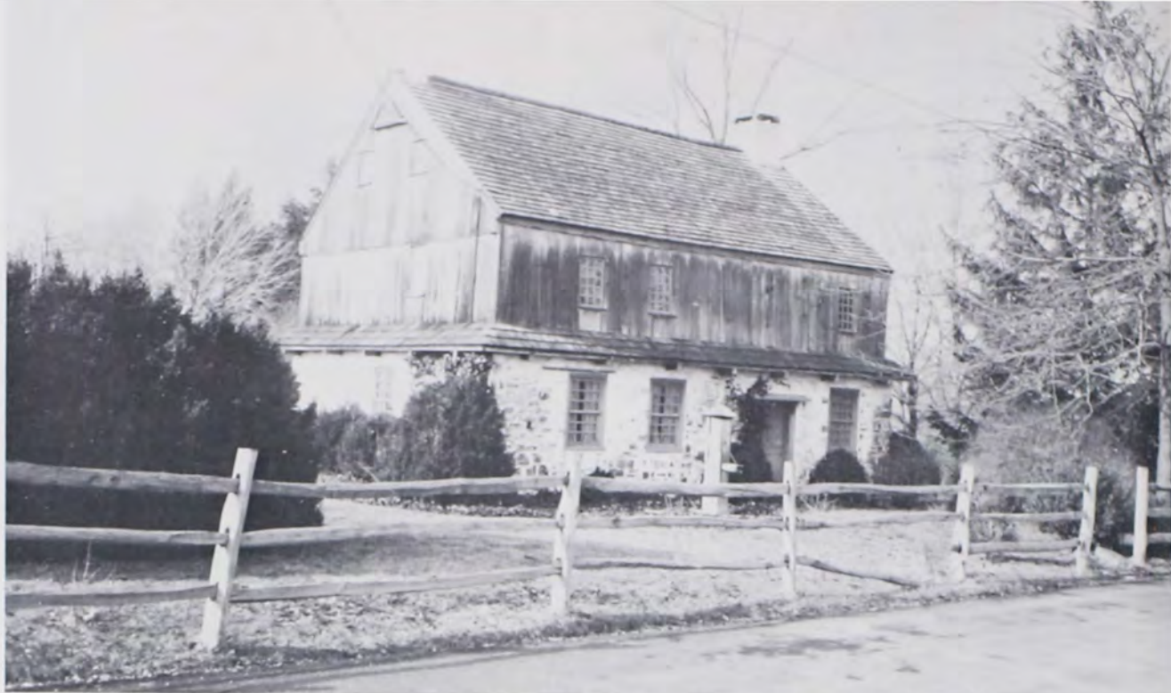
The Valentine Nungesser House, built circa 1730, Old Goschenhoppen, restored by Mr. and Mrs. Arthur Sullivan, a fine example of restoration projects done by private members. The Sullivans are now working on their second restoration—a Swiss central-hall house, circa 1760, with original out-kitchen or "French kitchen" as local Dutch Mennonites of area called them.
