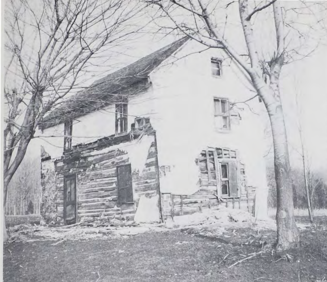
Valentine Nungessor house, dating from circa 1730-1750, is log on first story and half-timbered on second story. It stands on the same original tract as the Sullivans' house, which is log on second story, stone below. In process of restoration by Mr. Jack Levy, a member of the Goschenhoppen Historians Board of Directors.
