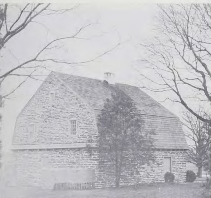
The Dielman Kolb House, Lederach, Pennsylvania, dating from about 1740—a Flemish Dutch Mennonite house being restored by Mr. and Mrs. Philip Detweiler, members of the Society.
