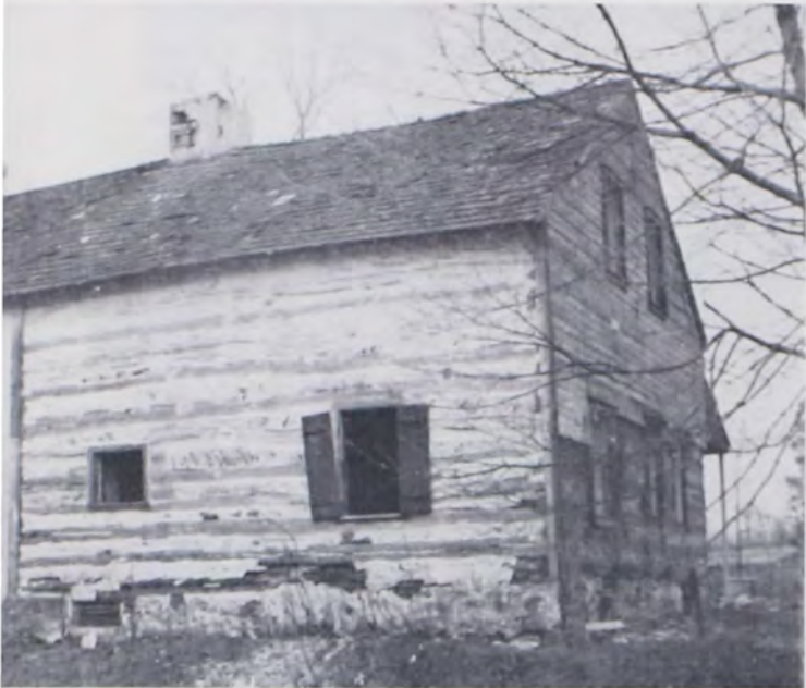
The Historians' First Project—removal of the 1755 Johann Frey Swiss-Mennonite log house from its site, threatened by the disease known as "galloping suburbia." It stood at the corner of Cowpath Road and Line Street, Lansdale, Pennsylvania, and is now reposing in "Jockeli" Lawton's barn, awaiting its eventual "resurrection morning" and restoration on a suitable site.
